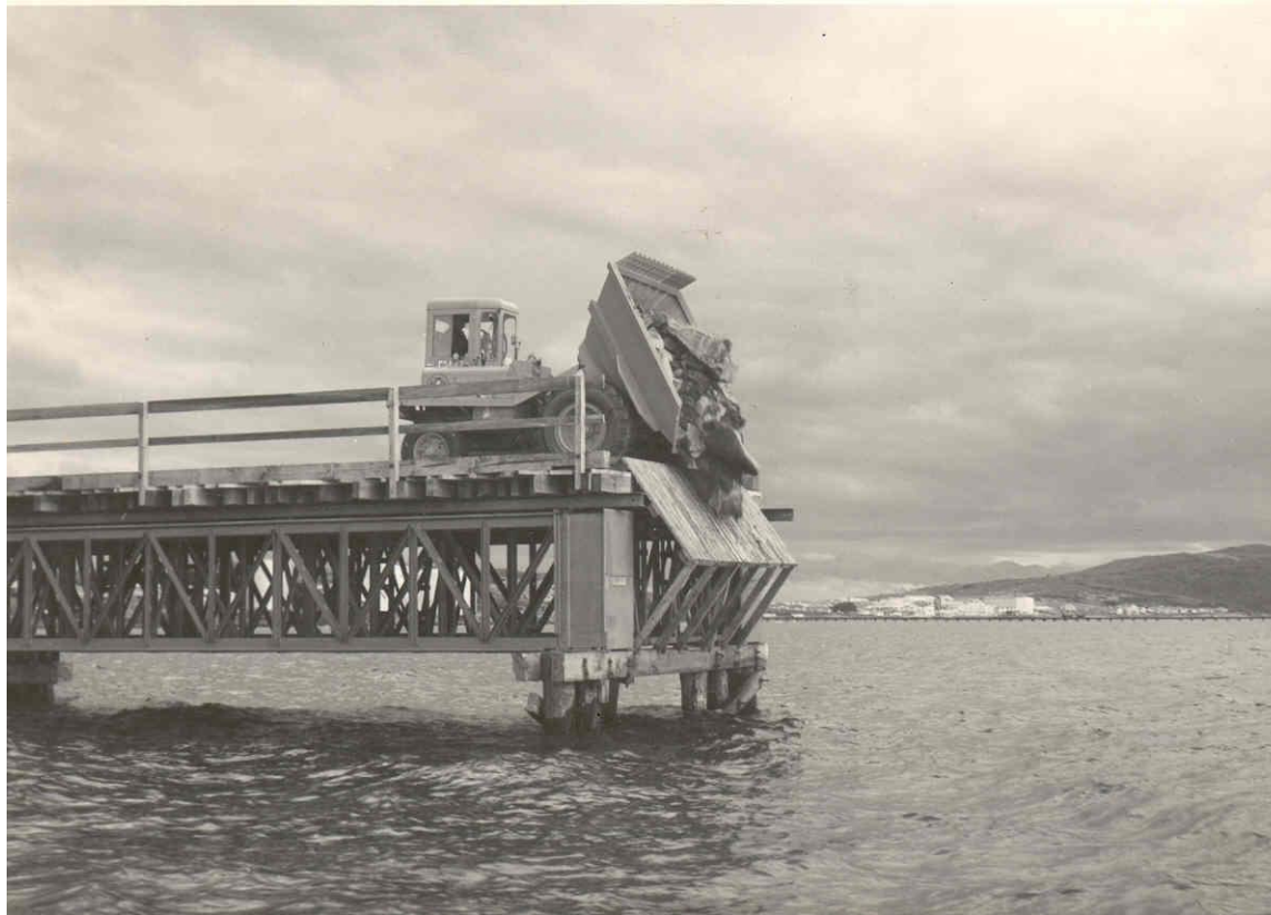
First dump of rock to commence retaining walls – 1956
