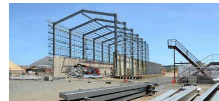
▶ The new Real Journeys building under construction.
