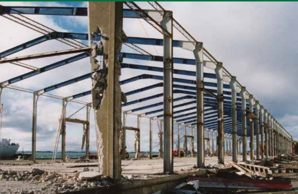
Number 4 cargo shed in the process of becoming a container terminal.
