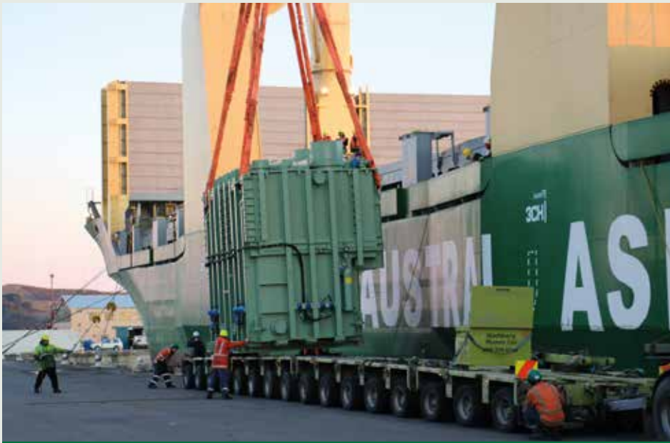
The transformer transformed from an item of ship-board cargo to a heavy load for road transport.
