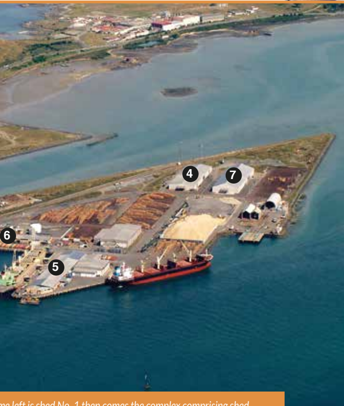
From left to right is shed No. 1 then comes the complex comprising shed No. 2 and Harbour cold stores adjacent, shed No. 6 is across the head and the recent additions, shed Nos. 4 and 7.
