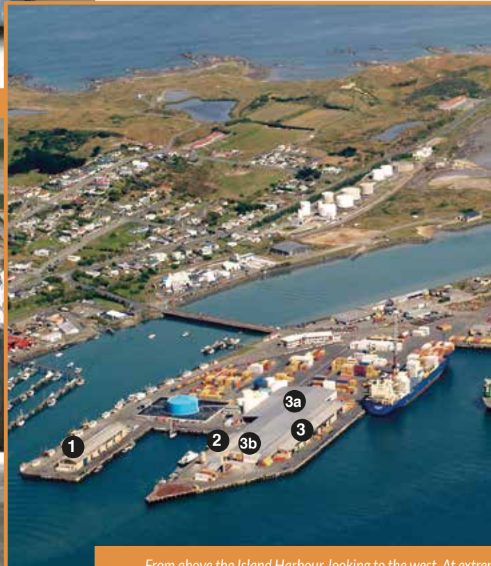
From above the Island Harbour, looking to the west. At extreme left is shed No. 1. At the top of the image are sheds Nos. 2, 3, 3A and 3B. Across the basin is shed No. 5 with the Island of the basin and beyond the log and woodchip area.
