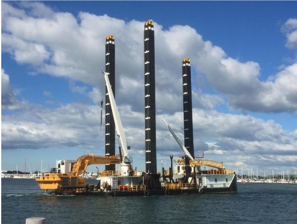
Caption: GPK De Donge 'B' Type Backhoe Dredger, to be operated by Heron Construction Company Ltd, throughout the dredging.
